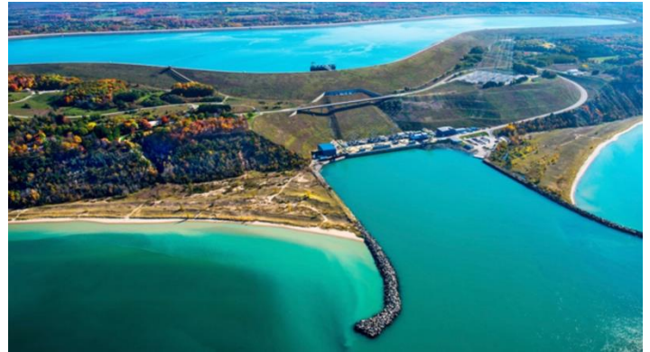
Image of Ludington Pumped Storage Power Plant
