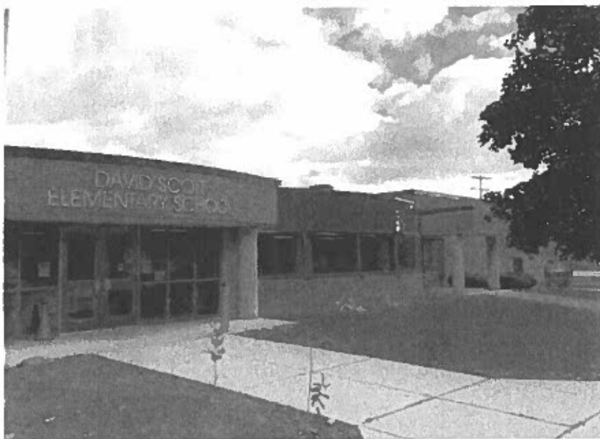
David Scott Elementary School in DeWitt. State environmental regulators fined a contractor overseeing renovations $15,000 for an asbestos release. (Photo: Craig Lyons)
