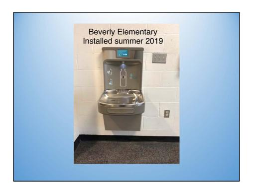
There is evidence that we can get this right. Here is a standalone, integrated filter station that was installed on the second floor of my kid's elementary school. When Birmingham sampled all the newly installed filter stations, every single station did not detect any lead in any filtered sample.
