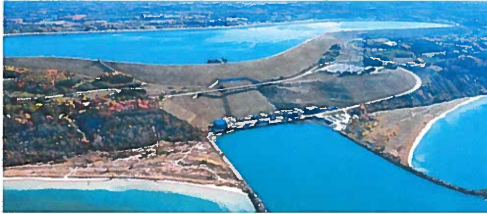
Ludington pumped storage facility
